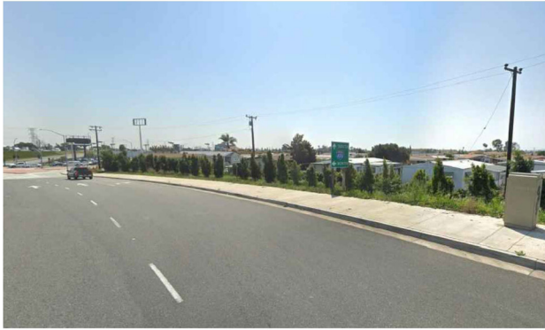
VIEW ON 405 FWY OFF-RAMP LOOKING SOUTHEAST 5
