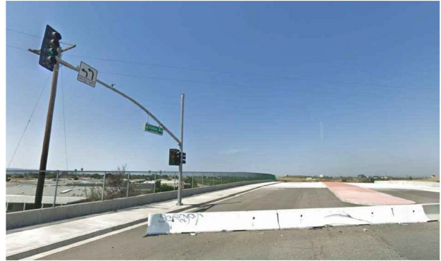
VIEW ON 405 FWY OFF-RAMP LOOKING WEST 6
